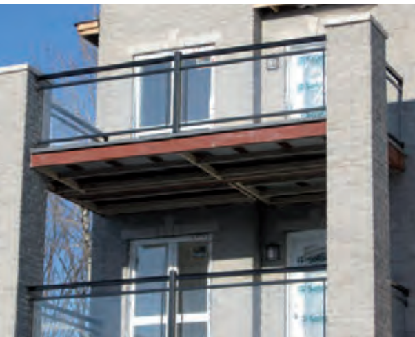
COLONIAL TOP RAIL WITH OPEN MID-RAIL AND 1/4" TEMPERED GLASS
