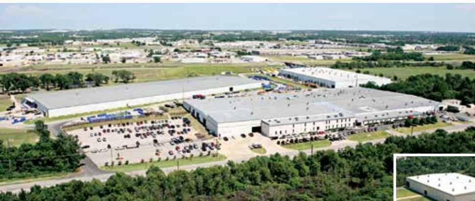
Ameristar's world headquarters, manufacturing & coil processing facilities in Tulsa, Oklahoma, USA.
